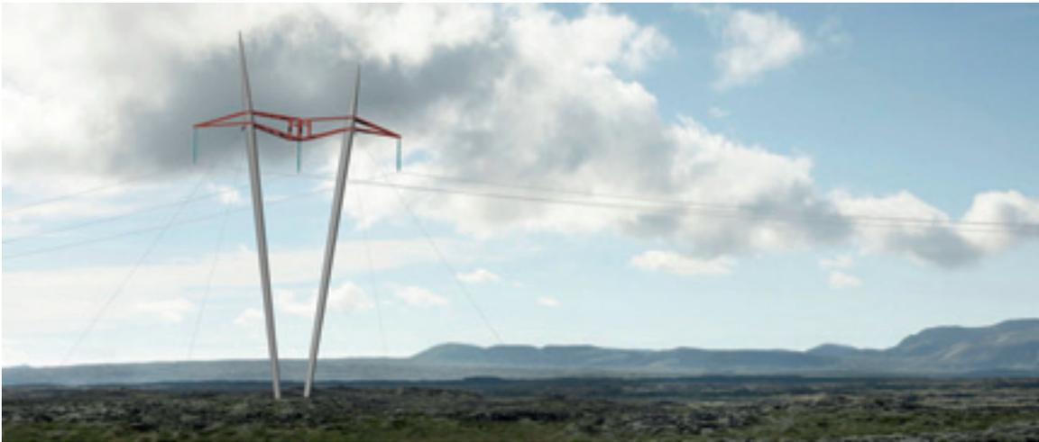
Another transmission tower design is “the Bird”, which was also submitted in the international competition. This design has also entered production and is scheduled to arrive in Iceland for installation in 2016. The Bird is a guyed tower with two tubes and a crossbar that resembles the wing of a bird – hence the name.
